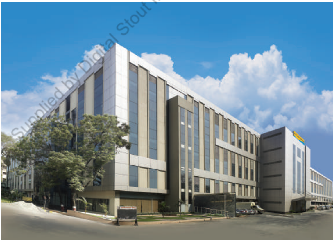
Switchgear Factory, Mumbai
