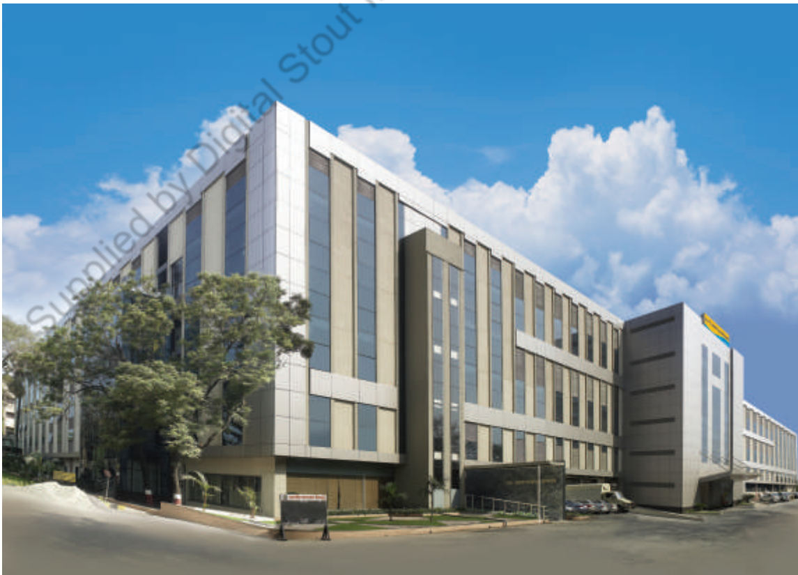
Switchgear Factory, Mumbai
